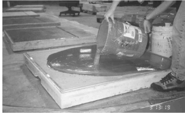
Figure 6 - Placement of leveling mortar
